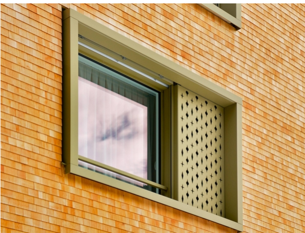
In detail: part of the larch wood facade
