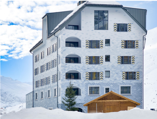
Heavy-duty roofs: Timbatec planned the roof structures
