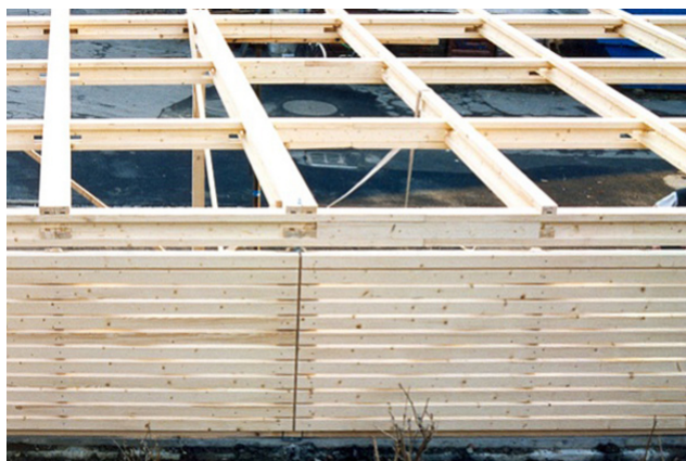
Finished car shelter
