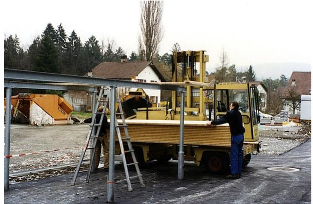
The architects envisioned a wooden slab laid over two steel girders - with a span of 4.50 meters. The plate was to be no more than about 4 cm thick and covered with greenery. This was not feasible, because with a construction less than 110 mm thick, the deflection would have been too great. But such a thickness would have been neither aesthetically nor economically satisfactory.
