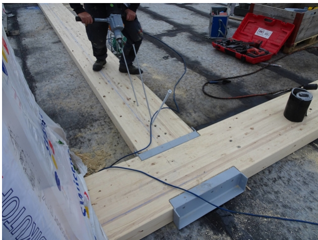
Reinforcement from above
