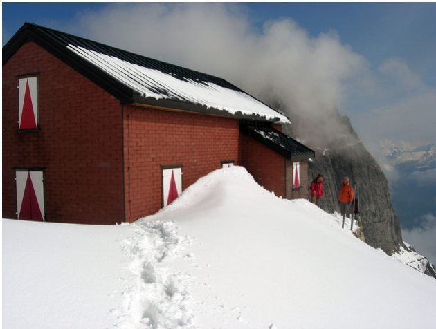
The original Dossen hut
