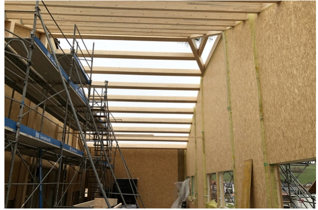
Extension gable side
