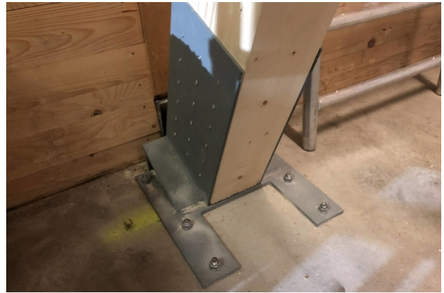
Strut connection bottom
