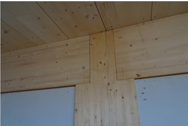
Bearing of the beams on the supports
