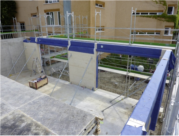
Under construction: first the wooden elements were installed, then the ceilings were concreted
