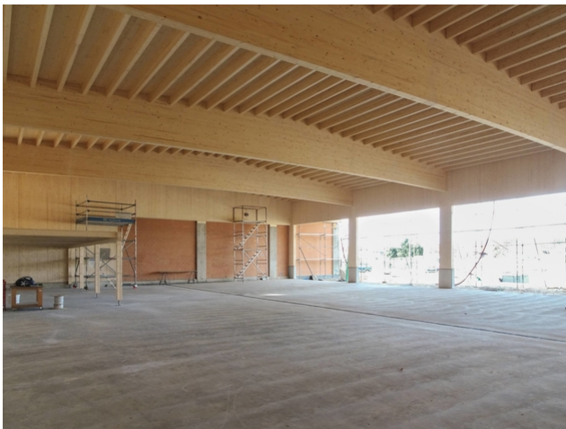
View inside: The 25 meter long trusses support the hall roof
