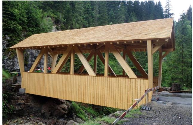
The bridge connects the districts of Sense and Gruyères and received a certificate for the use of Swiss wood. The new truss structure with shingle roof replaces the old Höllbach bridge, which was destroyed by arson in 2013.
