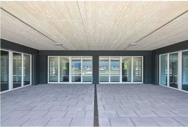
Entrance area with wooden ceiling
