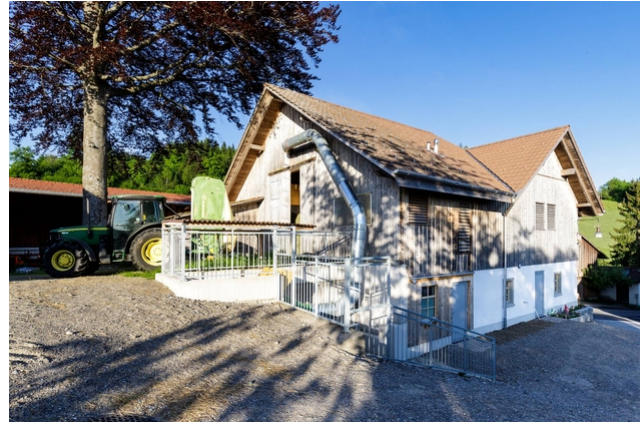
Exterior view of barn renovation
