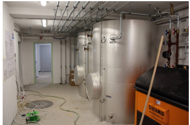
Building technology and building envelope are coordinated.
