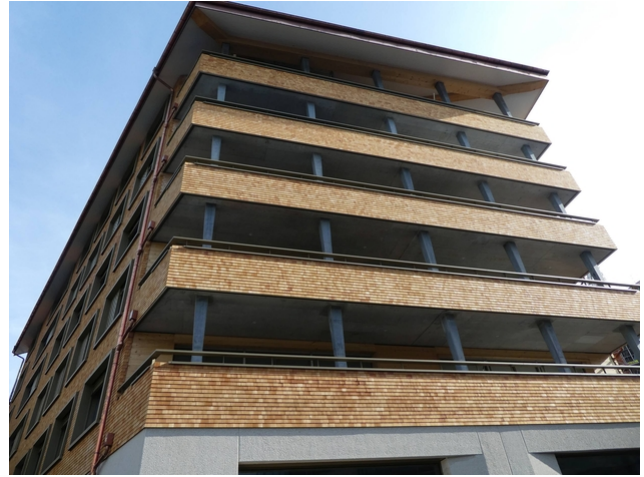
Wolf Apartment Building: Covered with wood shingles from top to bottom
