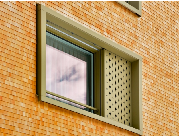
Close-up: Part of the larch wood facade
