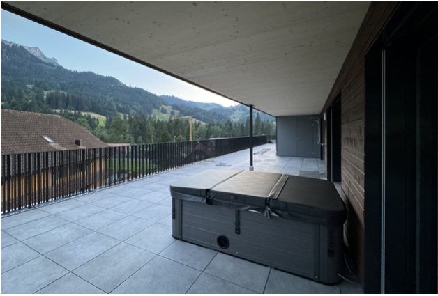
Continuous TS3 floor slabs. Terrace with views of the magnificent mountains of Entlebuch.
