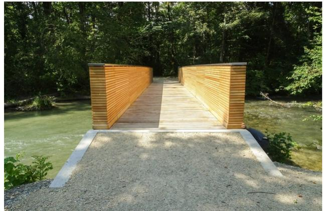
A new bridge in Lyss should be wider than the old one and passable for bicycles. Nevertheless, it will be supported by the existing abutments.
