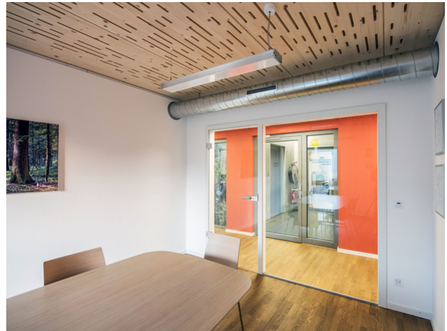
Feature: Lignum ceiling elements with acoustic holes
