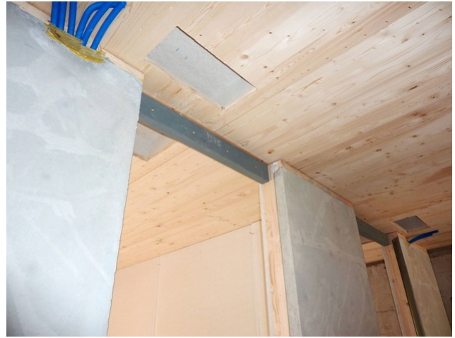
Wall coating as a heat accumulator
