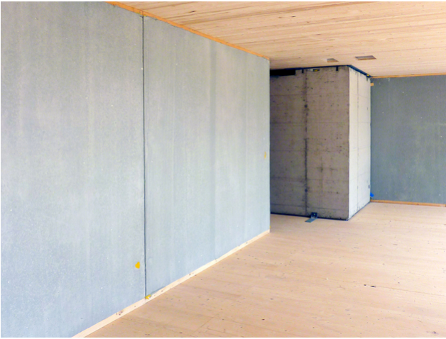
View wood concrete wall
