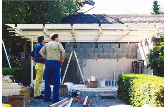
The client was looking for a solution for the roofing of their seating area. They wanted a more unusual solution than purlins and rafters. The situation allowed 2 line supports on 2 masonry walls at right angles to each other and a point support on a pendulum support.
