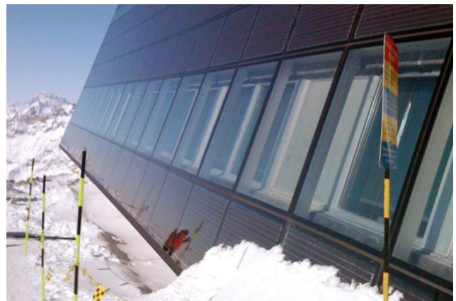
Facade with photovoltaics
