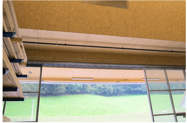
Sliding gate under the office wing - 15 m cantilever with minimum deflection
