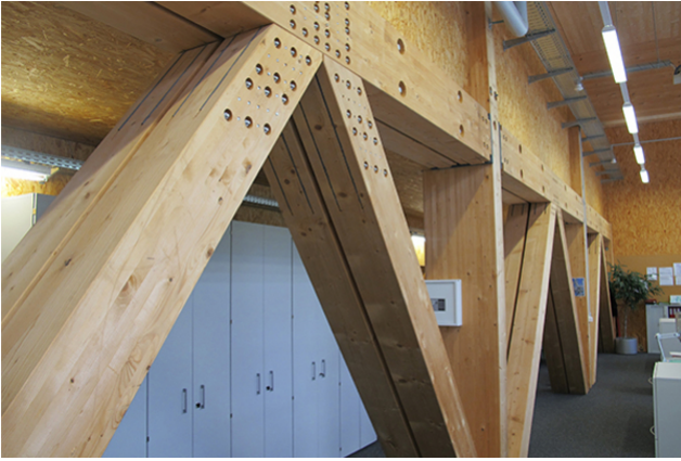
Truss in office wing
