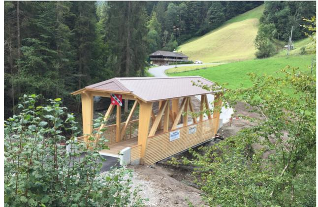
The new wooden bridge connects the two Bernese villages of Horrenbach-Buchen and Teuffenthal near Thun and replaces an old concrete bridge. The new crossing is capable of carrying loads of up to 32 tons.
