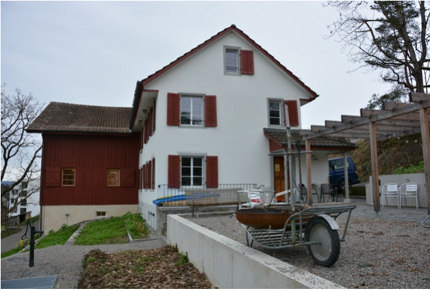
Exterior view QuarTierhof
