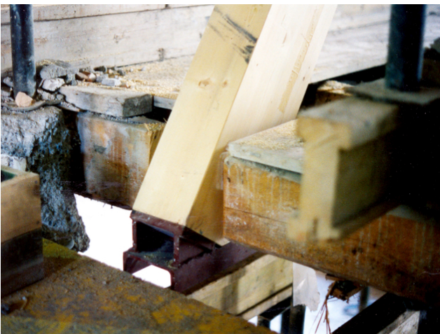
UNP beam, end support truss
