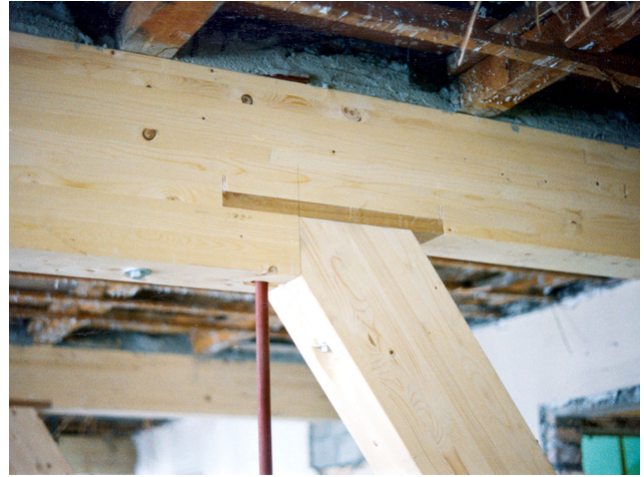
Transverse compression reinforcement with hardwood
