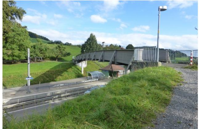
The pedestrian bridge near Vechigen was built in 1999. From the outside it was in relatively good condition, only the upper covers of the main girders seemed weathered and damaged.
