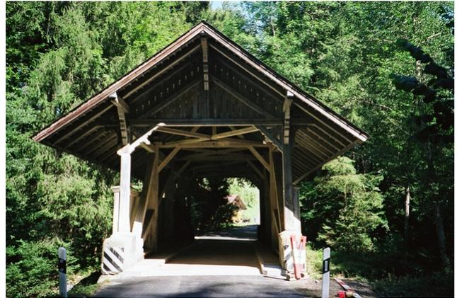
On behalf of the Civil Engineering Office of the Canton of Bern, the task was to assess the condition of the Lower Schwand Bridge, to prepare a rehabilitation concept and to supervise the rehabilitation on site. Furthermore, the 133-year-old bridge was to be largely preserved and integrated into its surroundings.
