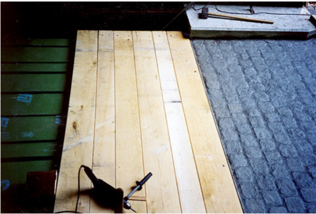
New roadway crossing
