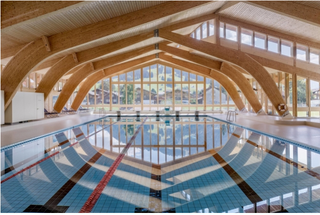
Impressive dimensions: supporting structure of the indoor swimming pool
