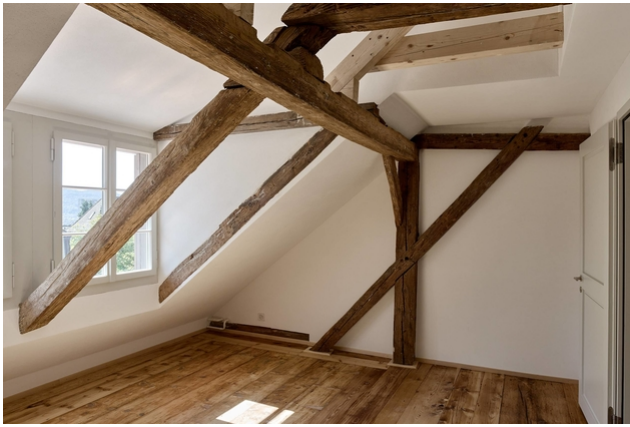
Existing roof truss
