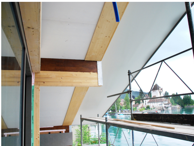
Garden hall with box beam ceiling
