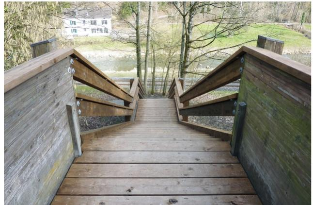
Large parts of the Horgen pedestrian bridge over the Sihltalstrasse had to be replaced. Many central wooden elements of the crossing were in poor condition.
