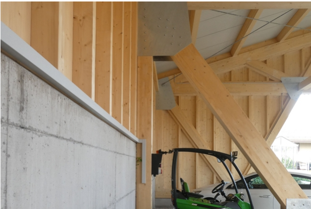
View of the truss structure of the timber frame
