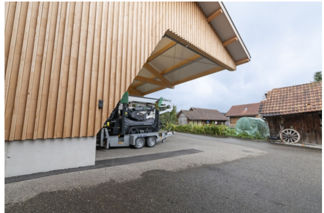
Roof structure with a long overhang
