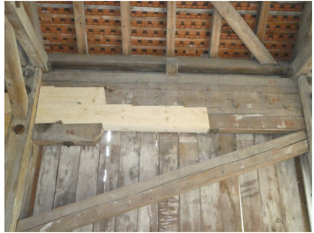
Existing and refurbished structure
